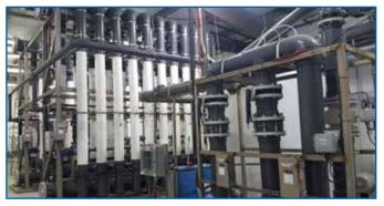
Two skids each using twenty X-Flow Membrane Elements (image courtesy of BioprocessH20).
